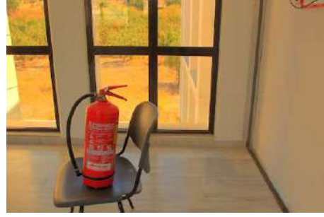
(b) Fire Extinguisher.
