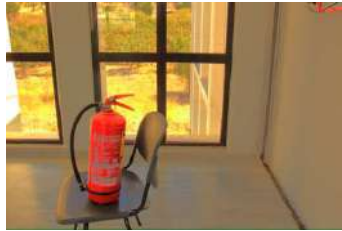
(b) Fire Extinguisher.
