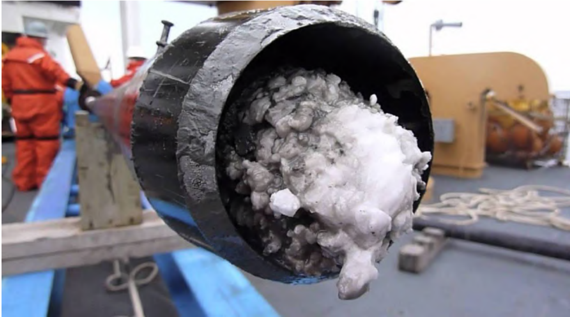
Figure 1.1: An example of a clogged line due to the hydrate formation. Image taken from TECPETRO.
