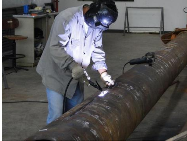
Figure 6: Covering of the gouged areas with Shielded Metal Arc Welding
