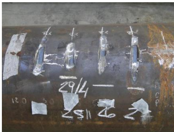
Figure 4: Gouging of the pipe to insert artificial defects in the welding region
