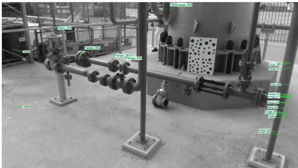
Figure 4: AR application of QuickVision in a refinery training plant. Assets that are not in view are represented in the image's border, pointing to their directions. From the image, it is straightforward to identify flanges 002, 003, 004 and valve 005.
