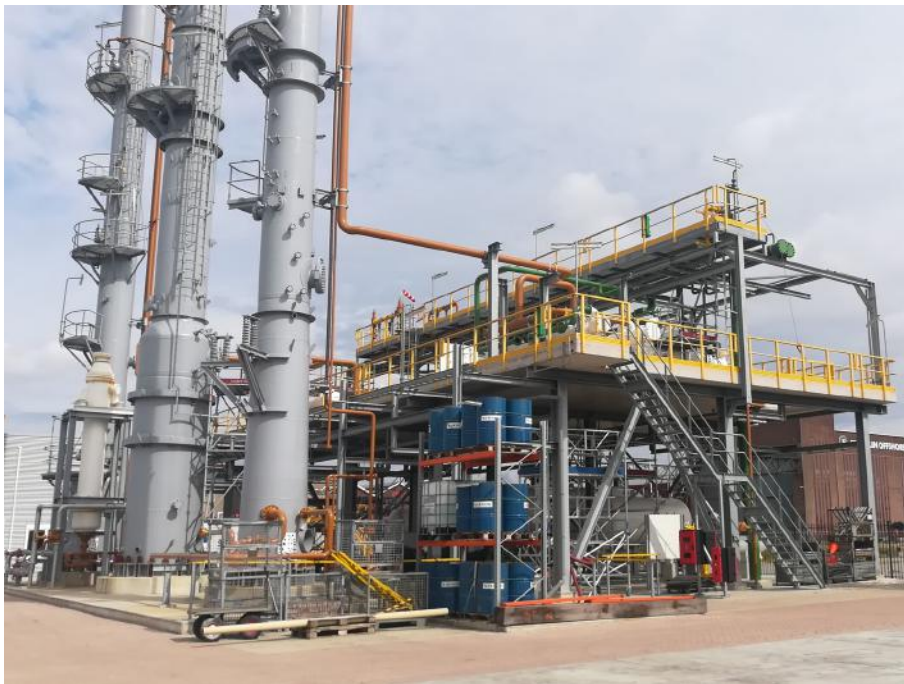
Figure 15: Refinery training plant overview.
