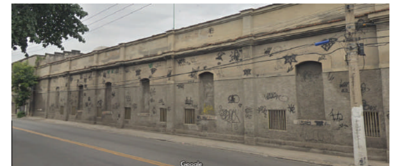
Fachada principal Rua Dr. March. 2018 Foto: Google street view
