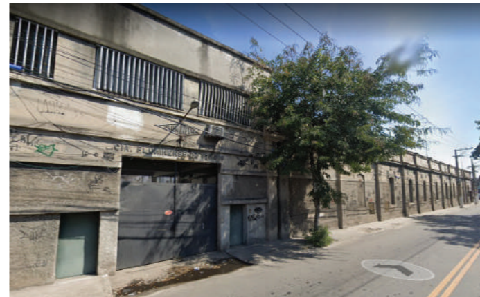
Fachada principal Rua Dr. March. 2019 Foto: Google street view
