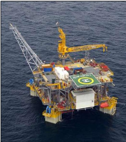
Figura 1-1 – Plataforma TLP (*Tension Leg Platform*) (MODEC, 2015).
