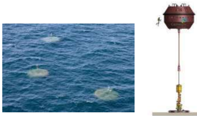
Figure 2-10- CETO5 wave energy converter 1
