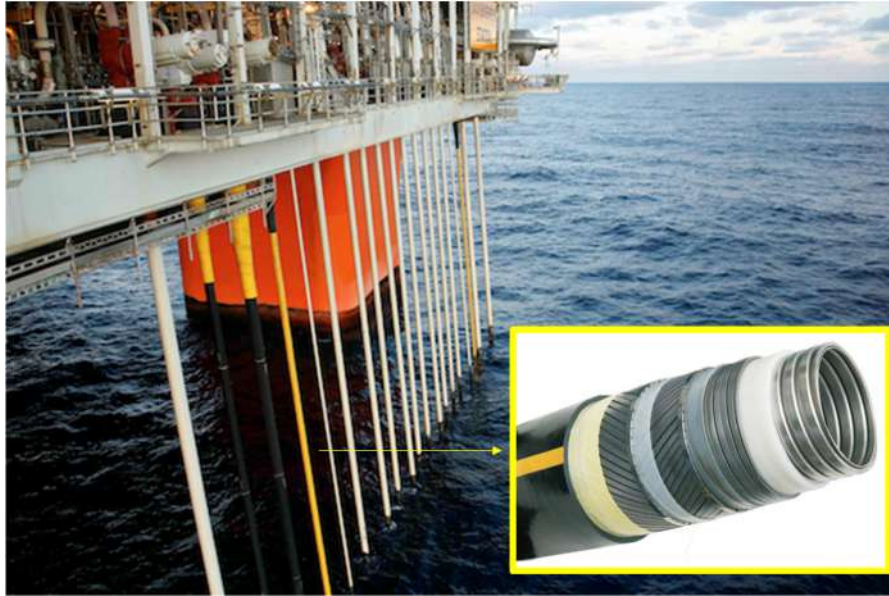
Figure 1.5. Flexible Pipe in operation (adapted from (SUBSEA WORLD NEWS, 2017)).
