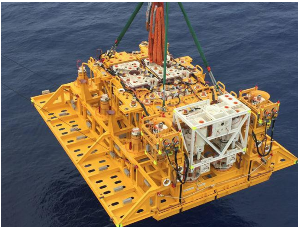
Figura 2.5: Manifold submarino equipado com mudmat (fonte: brazilenergyinsight.com ).
