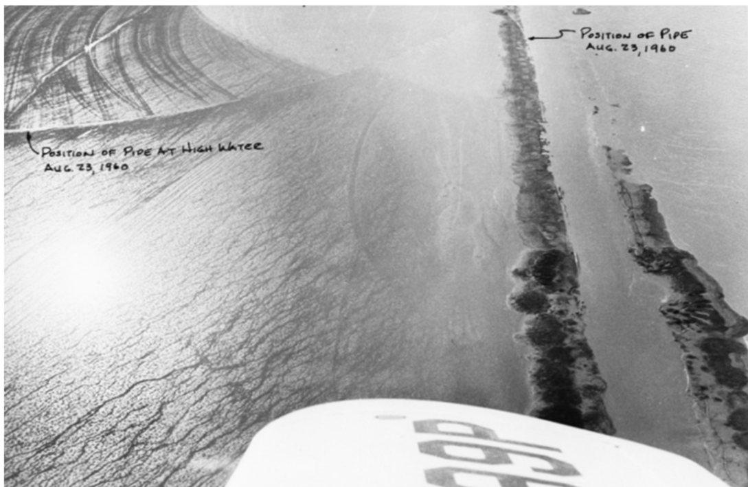
Figure 13 - Lateral Displacement of a Pipeline after a Storm. [13]
