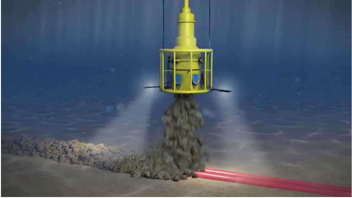
Figure 21 - Rock Dumping – Offshore fleet [20]
