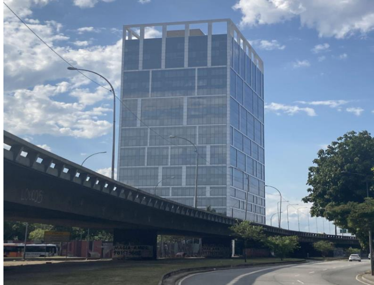
Figura 3 - Port Corporate Tower
