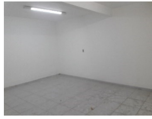
Figure 19: Restrooms before the refurbishment, 2016
