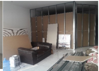
Figure 20: Front desk before the refurbishment, 2016
