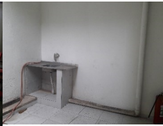
Figure 18: Coffee shop before the refurbishment, 2016
