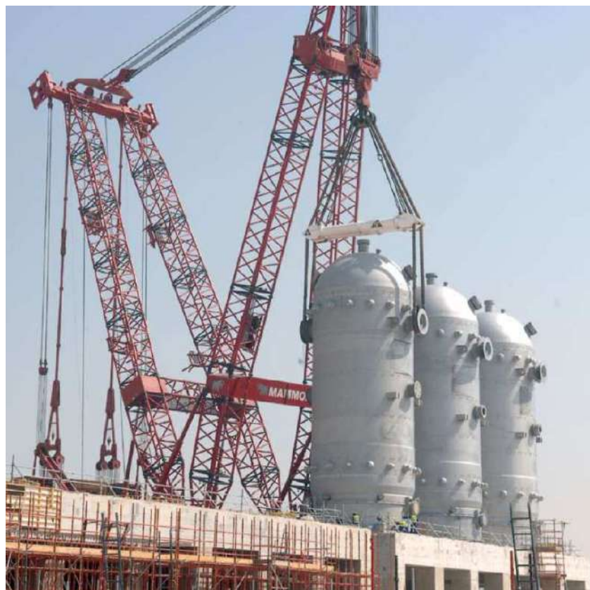
Figura 3.5 – Reatores HPS na Pearl GTL (SHELL, 2008b)
