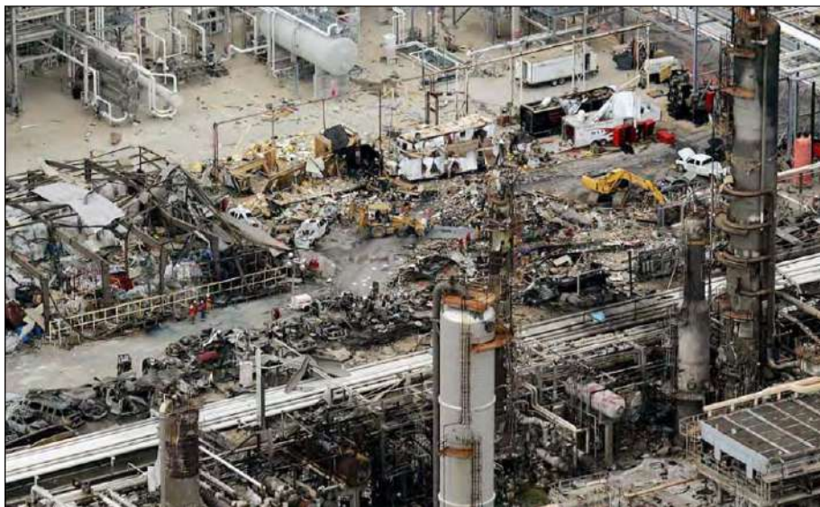
Figura 2.23 – Acidente na Refinaria Texas City.
