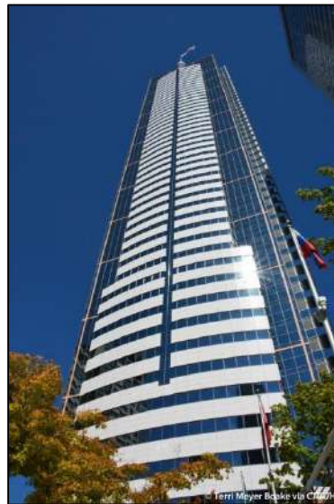
Figura 1-7. Two Union Square Building, Seattle, USA (BOAKE, 200-).
