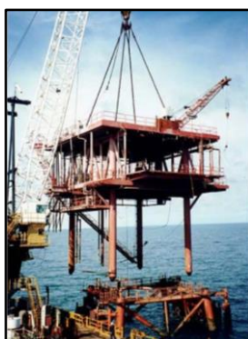
Figura 12. GA 189 Production Deck Lift.
