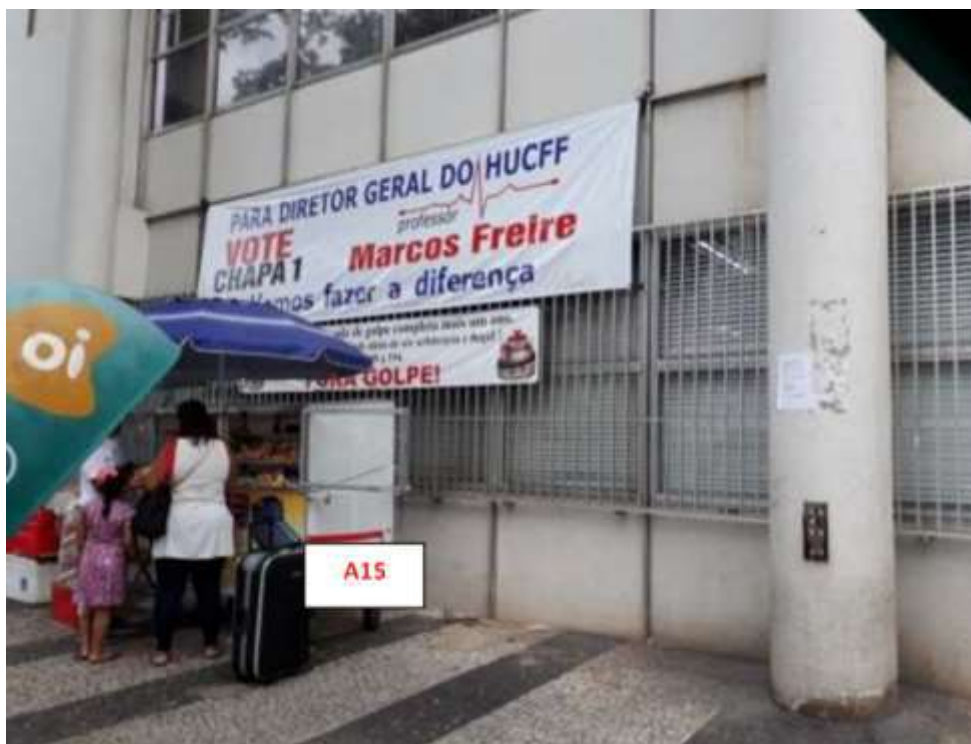
Fig.31. Rua Rodolpho Paulo Rocco – Portaria principal HUCFF (08.05.2019)
