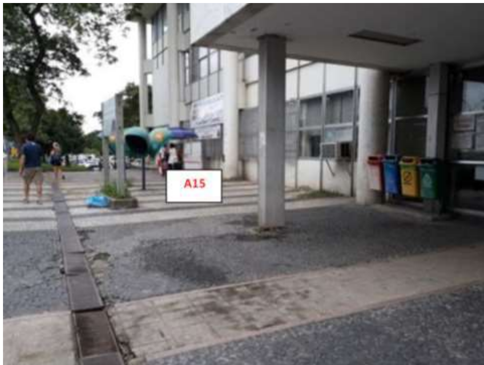
Fig.30. Rua Rodolpho Paulo Rocco – Portaria principal HUCFF (08.05.2019)
