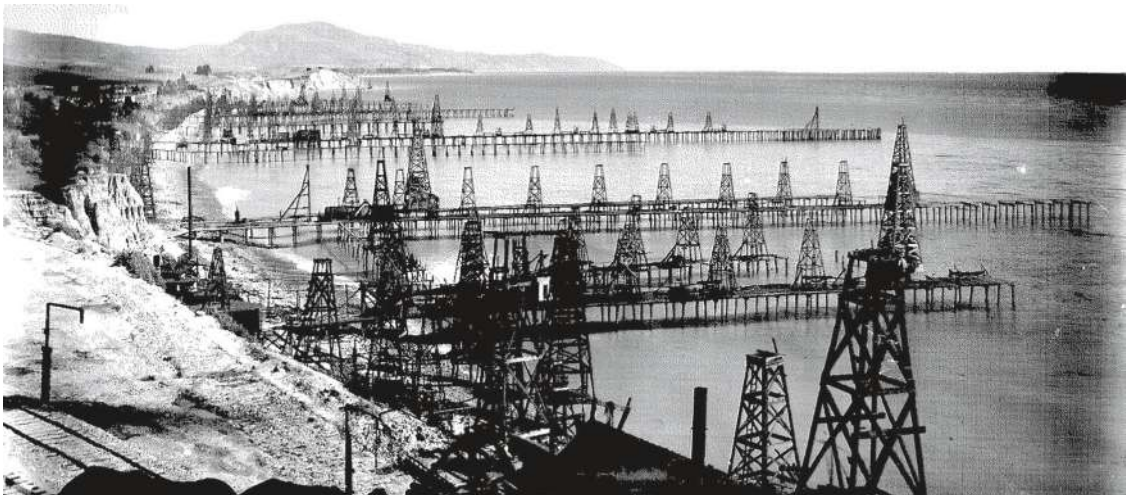
Figure 1.1: Piers and derricks at Summerland, California, 1901. (LEFFLER et al. [1])
