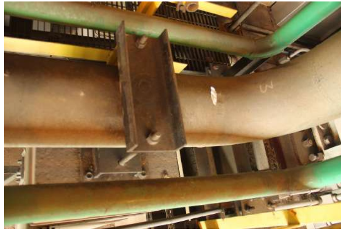
Figure 5.42: Intermediary pipe support.
