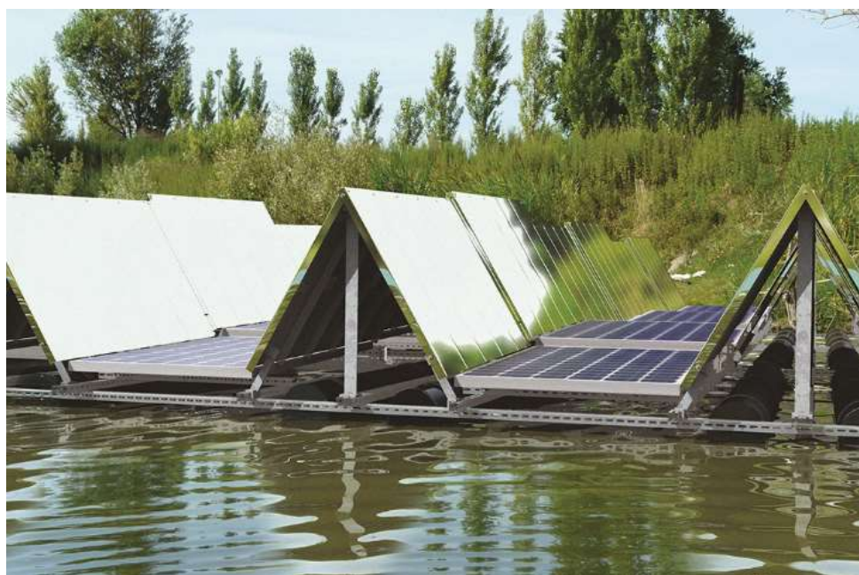
Figura 18: Modelo Italiano da Science Industry Technology (SIT) denominado Floating Tracker Cooling Concentrator (FTCC) (ROSA-CLOT; TINA, 2018c).
