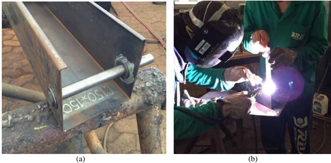
Figure 4.3 – Attachment of the washers in specimen holes: (a) positioning and (b) continuously TIG welding around the washer contour.
