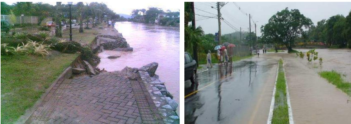
Fig. 39 (left): Signs of damages in the margins of Perequê-Açu (my photo) - point GPS 4
