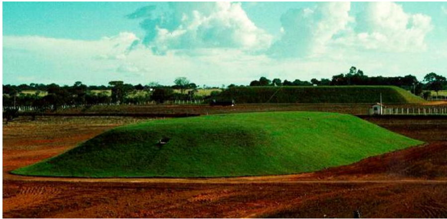
Fig. 1. View of the Goiânia near-surface repositories. The repository in the front contains relatively low-activity ^{137}\text{Cs} waste (specific activities less than 87 Bq/g), and the repository in the back higher-activity waste (specific activities above 87 Bq/g).
